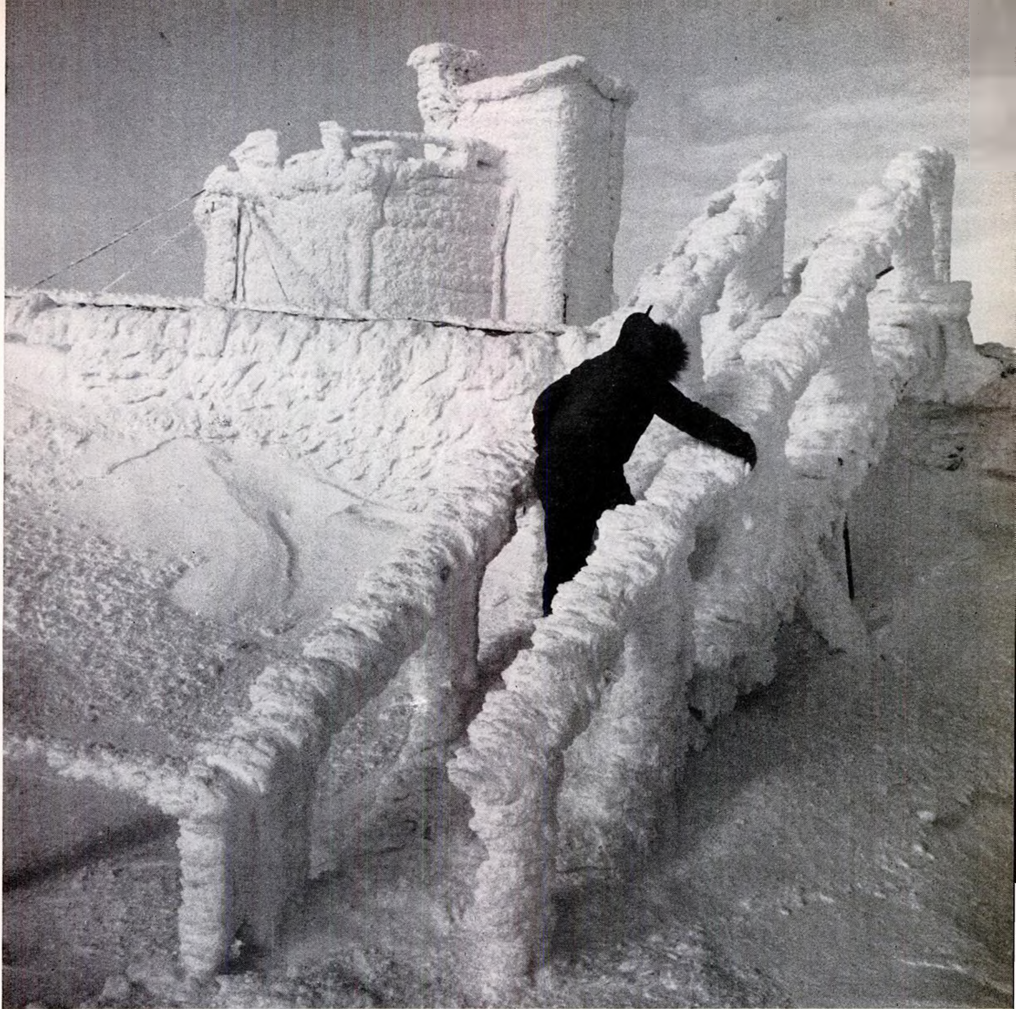
A TECHNICIAN CLAMBERS AROUND SUMMERTIME HOTEL WHICH, IN DEAD OF WINTER, STANDS CASTLELIKE AND FORBIDDING, ITS DOORS AND WINDOWS SEALED WITH FOOT OF ICE
