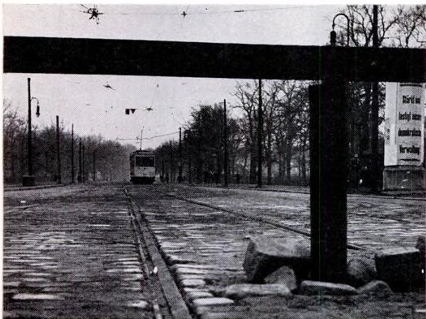
END OF THE LINE for Puschkin Allee tram is marked by Communists' recently erected fence of steel posts set in pavement with girder resting across top.
