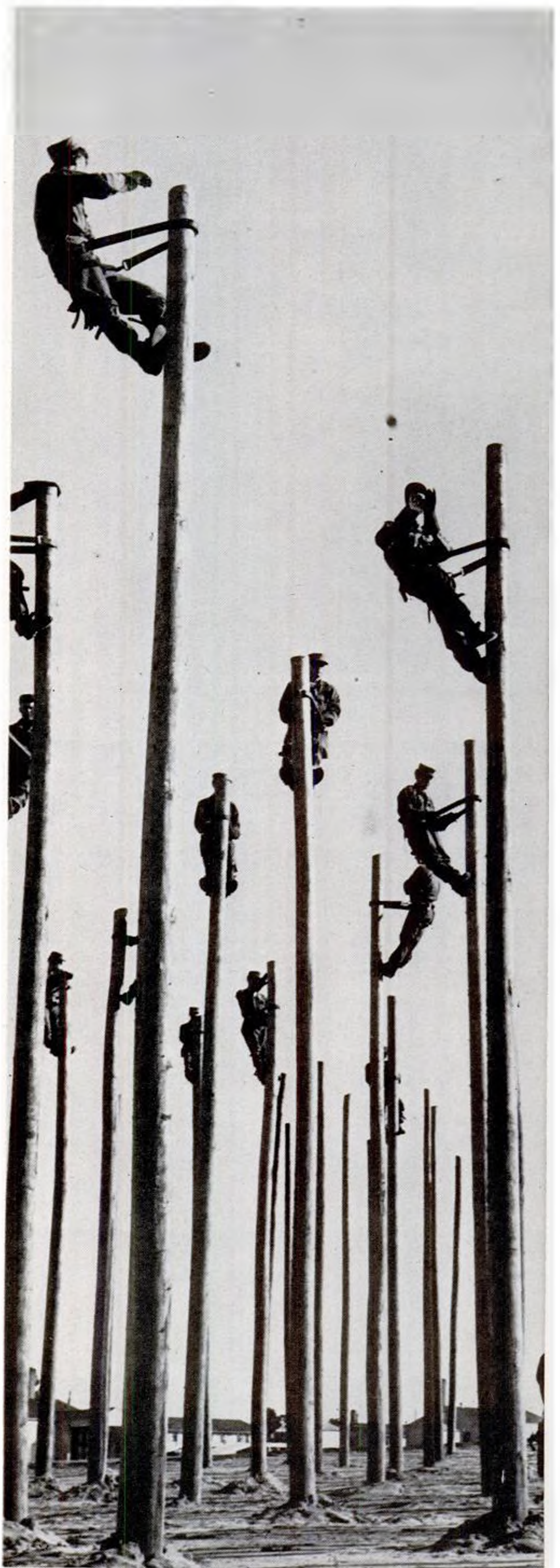
IN "POLE ORCHARD" Signal Corps trainees play catch with softball. Pole and telephone maintenance is part of Signal Corps work, and game atop 35-foot poles trains men to rely on their legs and belts, with hands free.
