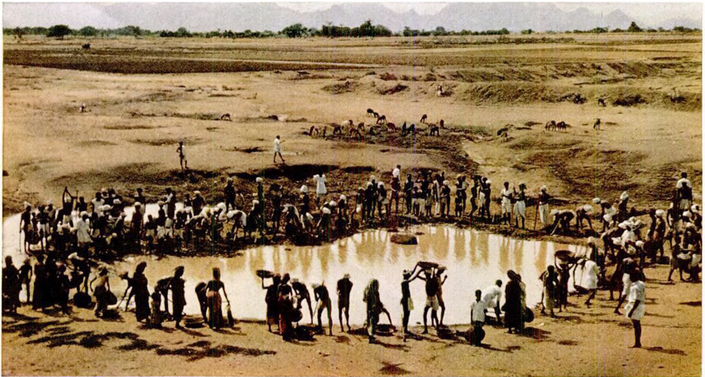
NEW WATER RESERVES , to be used in the drought seasons, are insured by deepening the bed of this village reservoir to increase its storage capacity.
